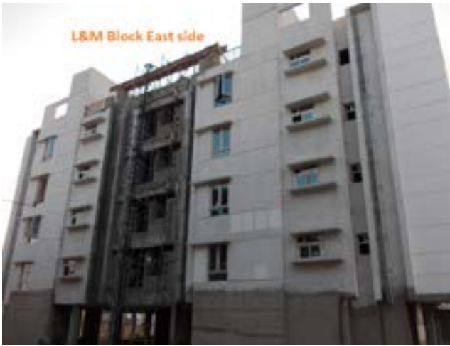
East Side of Block L & M
